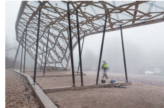
Image Credits: Design + Make, Timber Seasoning Shelter
