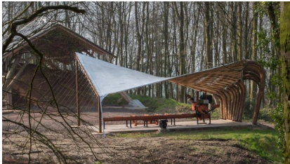
The completed shelter features steam bent logs supporting slender finger-jointed timber laths
