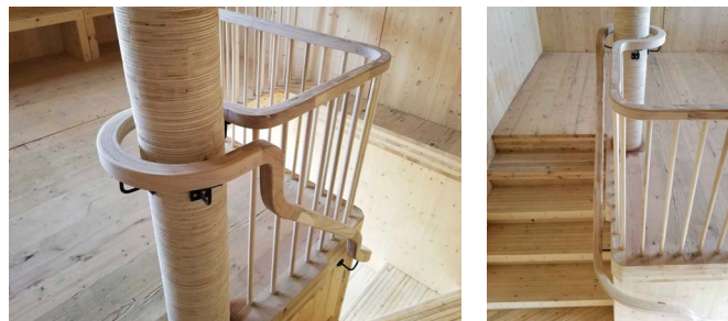
Steam bent curvy handrail designed and built as part of the South Sioux City Orchard Facility, a CLT structure in Nebraska. Project work done by students of University of Nebraska-Lincoln, led by professor Jason Griffiths
