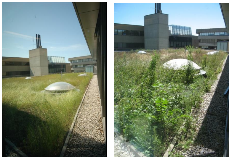
Figure 5 Arts and Administration green roof, University of Toronto, 2005 (left) and 2013 (right).
