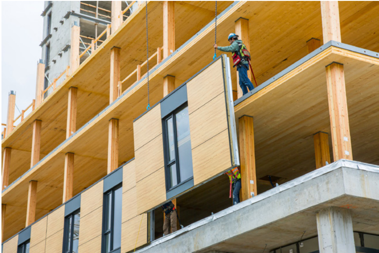
Large format panels with integrated windows and cladding. Detailing resembles curtainwall and/or precast wall systems technology spanning outboard of the floors. (Courtesy naturally:wood)
