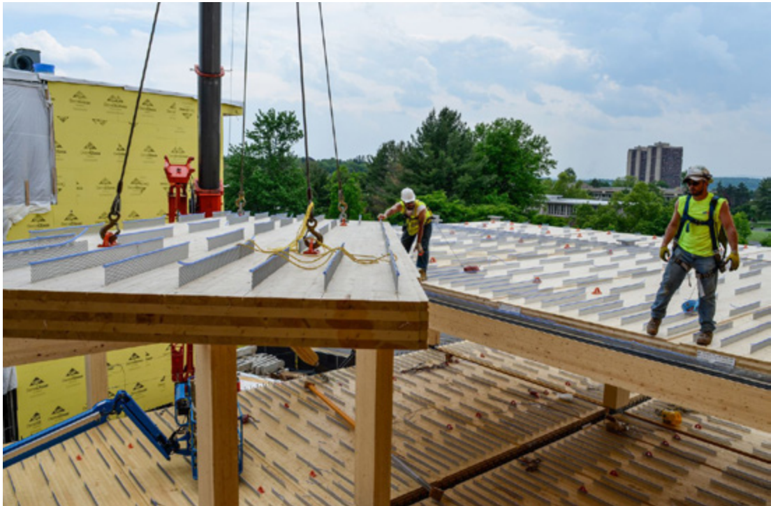
The efficient delivery and rigging (hoisting) of mass timber components is critical to gain the mass timber advantage. Efficient deployment of cranes and booms is an important erection strategy to optimize during the planning stage of a mass timber project. (Alex Schreyer/UMASS)
