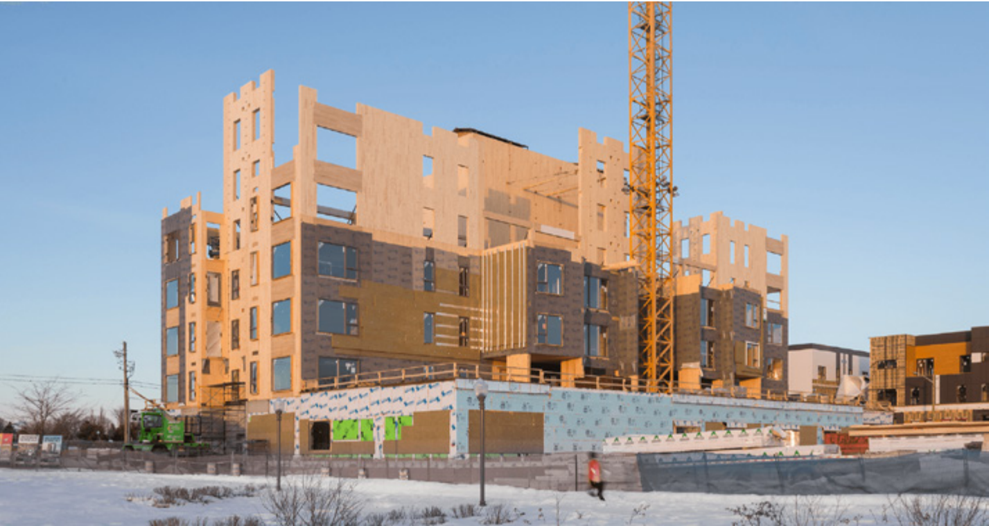
Mass timber panel systems are well suited to multi-unit housing projects. The Origne is a 12-storey, 92-unit timber tower situated on a ground level concrete podium. It features numerous innovations including a lateral load resistance system using cross-laminated timber panels. (Cecobois)
