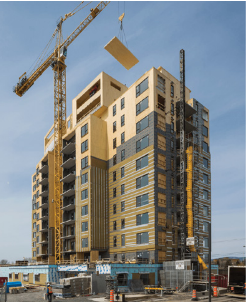
Mass timber panels save construction time. The wooden structure for the Origne project was erected in just four months. It was estimated that about a 25% savings in total project construction time resulted from selecting the mass timber panel structural system. (Cecobois)
