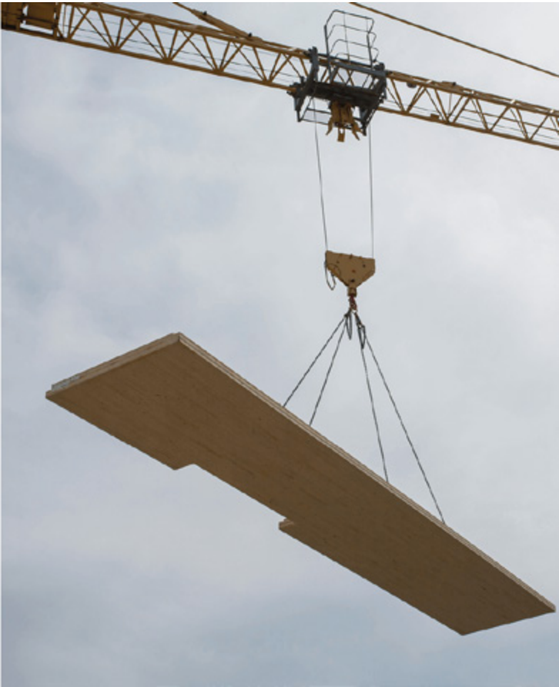
Mass timber panels save construction time. The wooden structure for the Origne project was erected in just four months. It was estimated that about a 25% savings in total project construction time resulted from selecting the mass timber panel structural system. (Cecobois)
