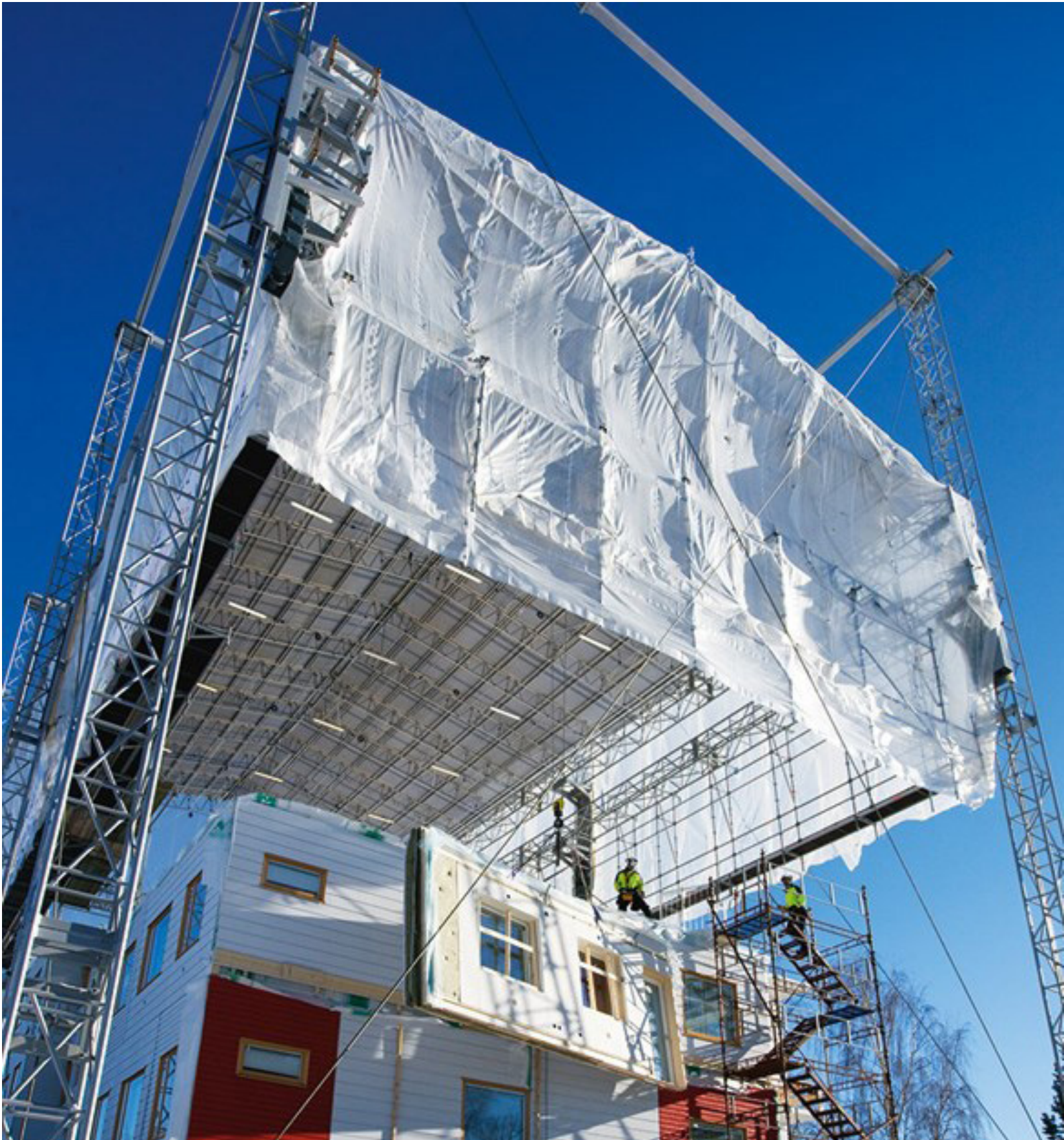
Construction safety and productivity are enhanced by proper moisture management practices. The installation of this prefabricated, panelized enclosure system proceeds on a year-round basis under dry site conditions. (Swedish Wood)
