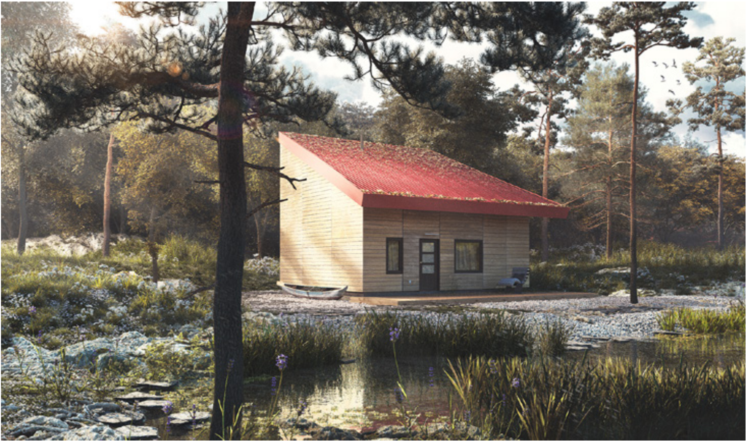
Mass timber for Indigenous communities. Cardinal House is a prototype for a prefabricated mass timber home intended to help meet the housing needs of First Nations communities. Designed by renown Canadian architect, Douglas Cardinal, and manufactured by Element5, assembled by MCH, the prefabricated, modular design and mass timber construction delivers a high-performance, durable home that can be passed down through the generations.
