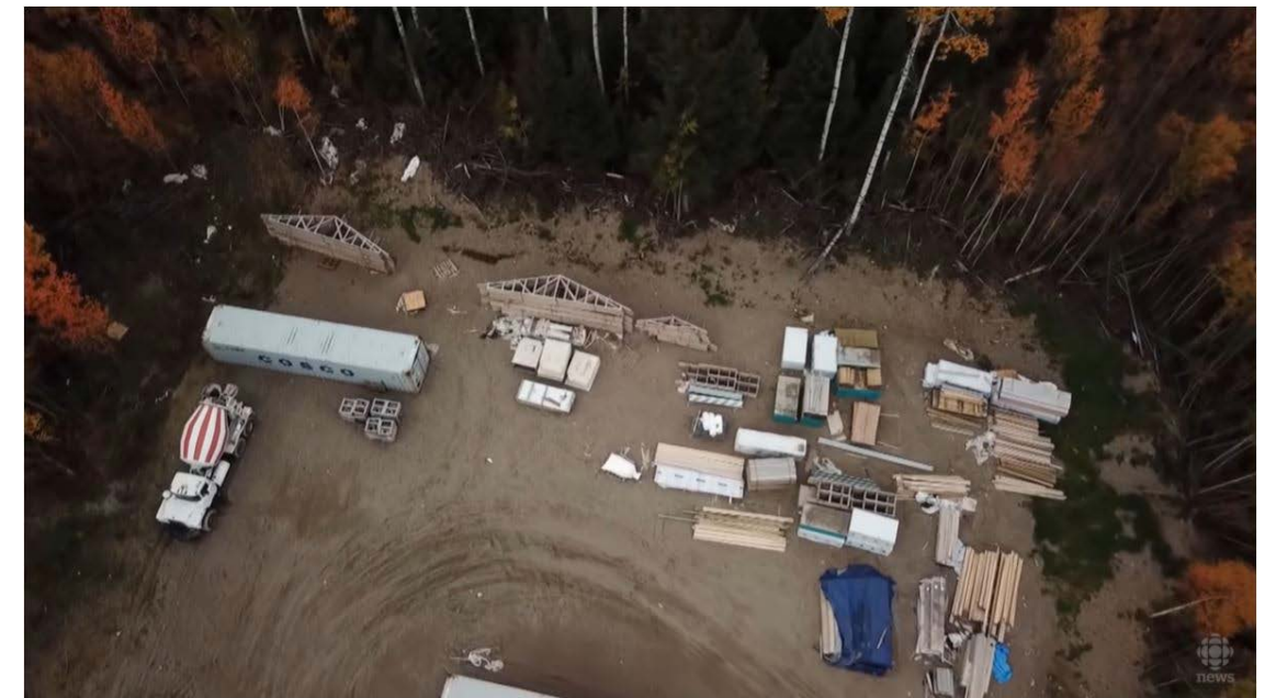
Material lays unused in Nibinamik as the First Nation experiences lengthy processes to acquire funding for construction crews. Image Credit: CBC News: The National.
