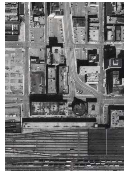
1969 Metro Toronto Planning Department, Air Photos. City of Toronto Archives. Series 12, Folder 1969, Item 28.
