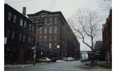
1988 Mowat looking south from King. Toronto (Ont.). Planning and Development Dept. City of Toronto Archives. Fonds 200, Series 1465, File 723, Item 5.
