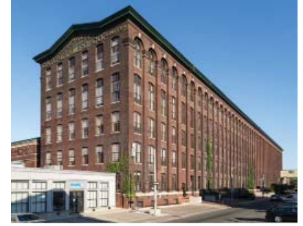
2016 North and west elevations of the former carpet manufacturing facility that runs the length of Mowat Ave. - The building has since been converted to office and commercial space. Vik Pahwa Fonds. City of Toronto Archives. Fonds 546, Item 59.
