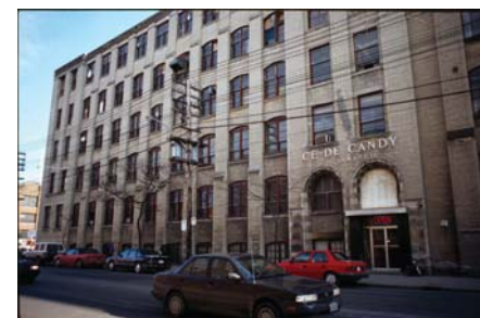
1983 Ce De Candy Company, south-east corner of Queen and Shaw streets. Toronto (Ont.). Planning and Development Dept. City of Toronto Archives. Fonds 200, Series 1465, File 430, Item 11.
