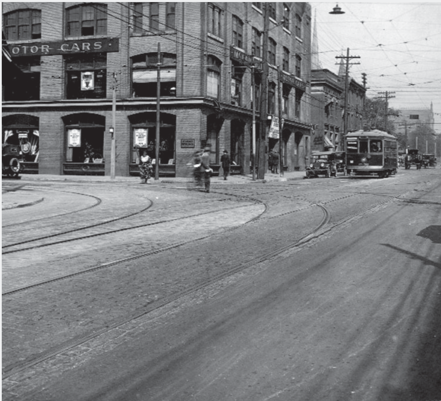
Richmond South Switch looking N.W. Aug. 31/23 (claims)
