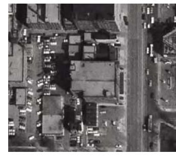
1967 Aerial photograph showing the parapet line between the two phases of construction. Metro Toronto Planning Department, Air Photos. City of Toronto Archives. Series 12, Folder 1967, Item 27.
