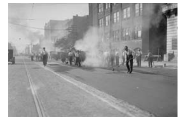
1928 West side Spadina Avenue, King to Adelaide streets - asphalt and bitulithic pavement. Dept. of Public Works Photographs. City of Toronto Archives. Fonds 200, Series 372, Subseries 58, Item 1203.
