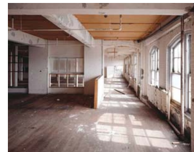
1984 Conversion of a five-storey factory structure into 120 residential lofts and amenity space; two levels of underground parking in the existing basement;
