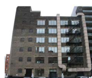
2022 North elevation with new and old glazing, a steel fire escape, and mechanical ducts. 10.2 - 468 King Street West. Heritage Impact Assessment. ERA Architects Inc. February, 2022, 27.
