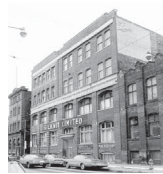
1973 1973 photograph showing the alterations undertaken by Silknit which relocated the door, removed the original door and many of the decorative stone elements. Figure 23. Intention to Designate, Ontario Heritage Act - 582 King Street West. Heritage Preservation Services. City of Toronto Archives.
