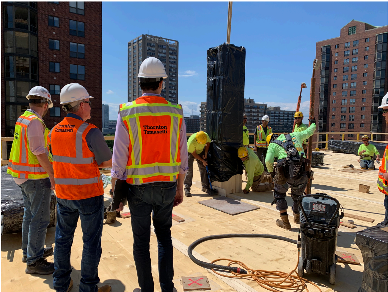
The installation of one of the tower's many mass timber columns. Photo courtesy Thornton Tomasetti.
