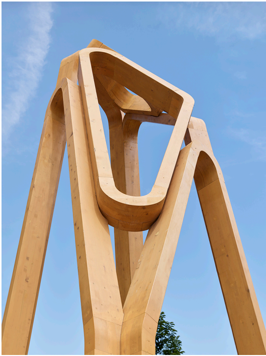
Custom joinery of Lodestar Tower's mass timber components. Image Credit: Andrew Latreille
