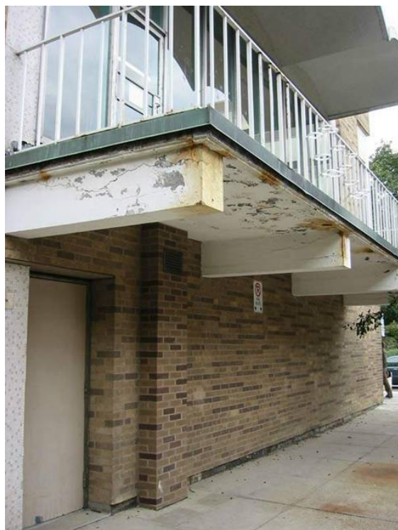
Figure 2 – A typical example of deferred maintenance on the St. George Campus where rehabilitation has the potential to improve durability and thermal performance.
