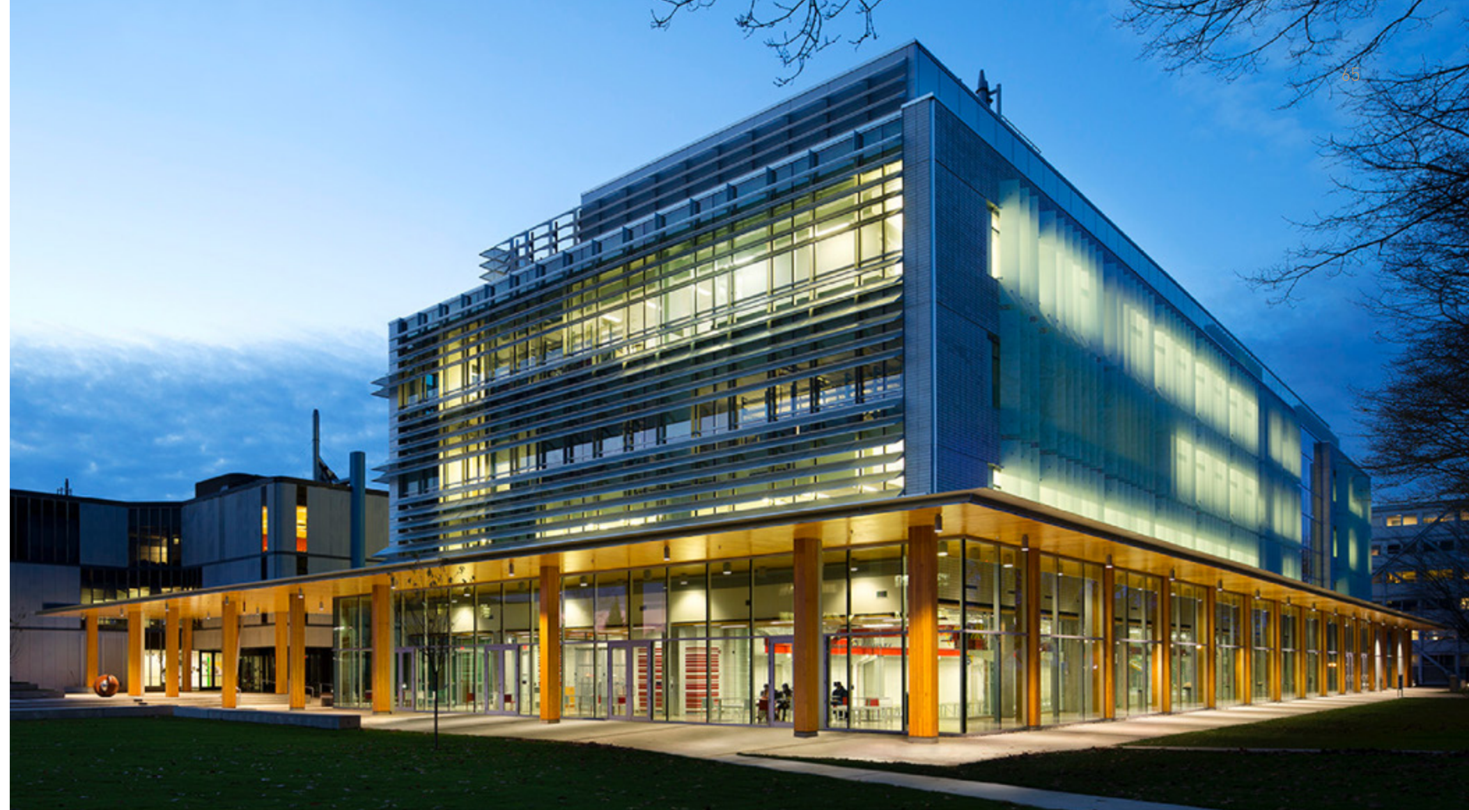
Mass timber innovation in support of sustainable natural resource education. The Earth Sciences Building, University of British Columbia is the one of the largest panelized wood building and among the largest applications of cross-laminated timber in North America. It is critical that institutions and organizations that wish to advocate the goals of sustainable development adopt wood as the material of choice in their facilities. (Perkins + Will Architects, Structurlam – Martin Tessler)
