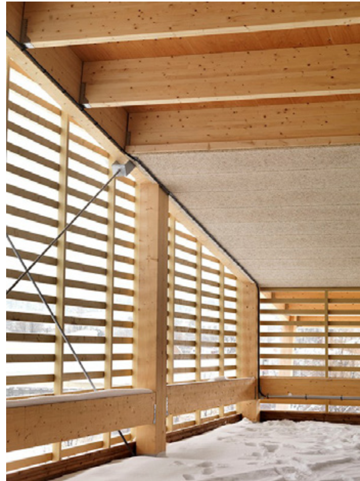
Four storey mass timber post and beam mixed use building. Located in Skellefteå, Sweden, this building features three storeys of parking on top of the ground level stores. The parking deck floors are covered with polyurethane to protect the cross-laminated timber decking from absorbing water. Generous overhangs and an open screen façade for ventilation ensure the drying potential exceeds the wetting potential on an annual basis to maintain a safe moisture balance. (Setra Group)
