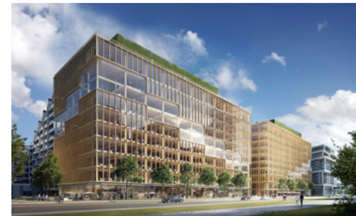
T3 Bayside by 3XN Architect, Denmark. This proposed development near Toronto's waterfront seeks to create a campus of two office buildings using mass timber building technology. According to the architects, the breathable and absorbent properties of wood allows for the release of moisture to ensure a naturally regulated, healthy indoor environment. (Hines)
