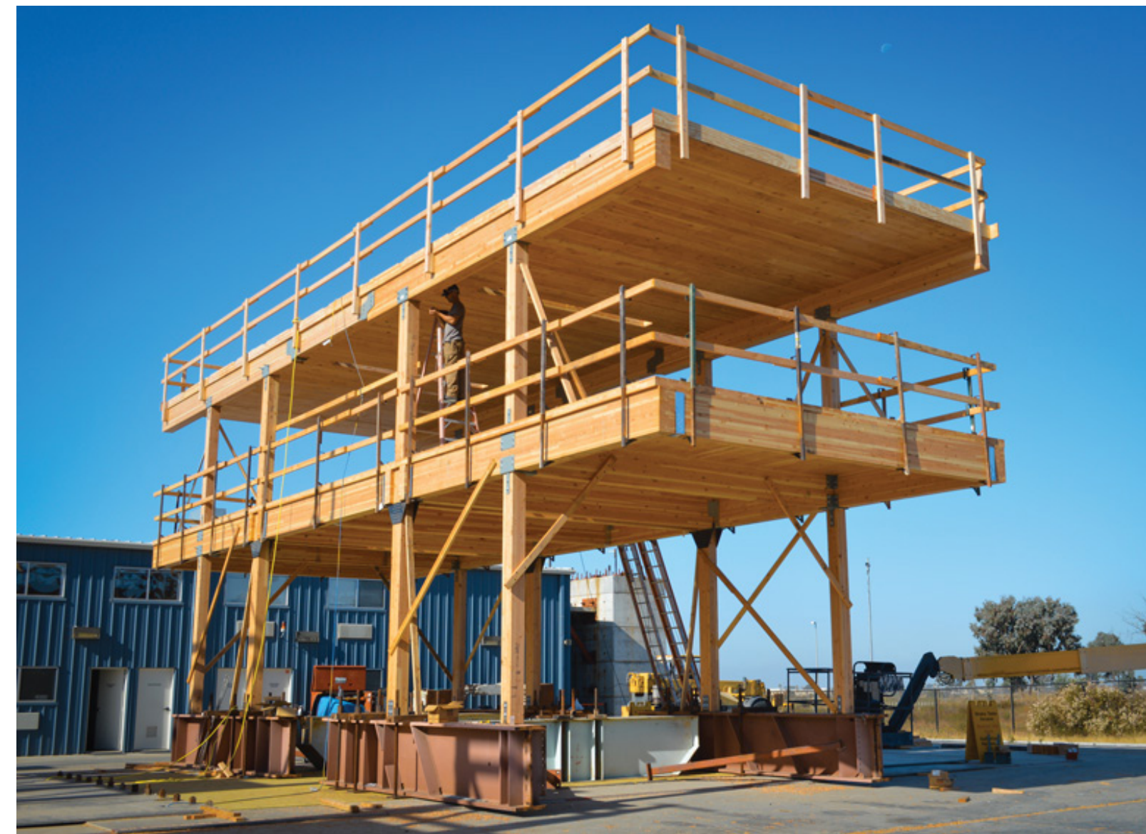
Full-scale seismic testing of mass timber. Testing of full-scale mock-ups on a shake table to assess lateral resistance is an ongoing global research effort as mass timber technical innovations develop new concepts, materials and connectors. Special testing of this kind may be required to confirm compliance for alternative solutions under building codes. (University of California, San Diego)
