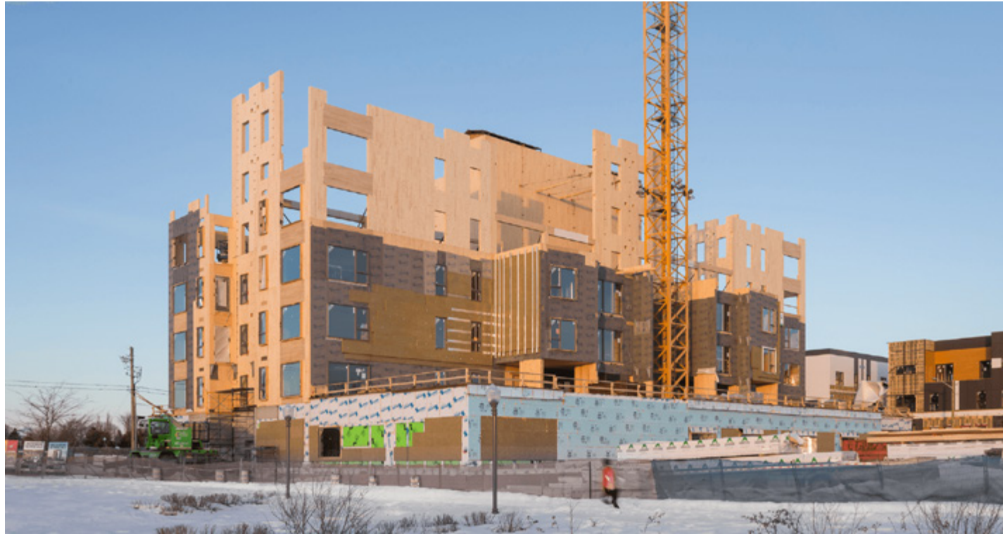
Mass timber panel systems are well suited to multi-unit housing projects. The Origine is a 12-storey, 92-unit timber tower situated on a ground level concrete podium. It features numerous innovations including a lateral load resistance system using cross-laminated timber panels. (Cecobois)
