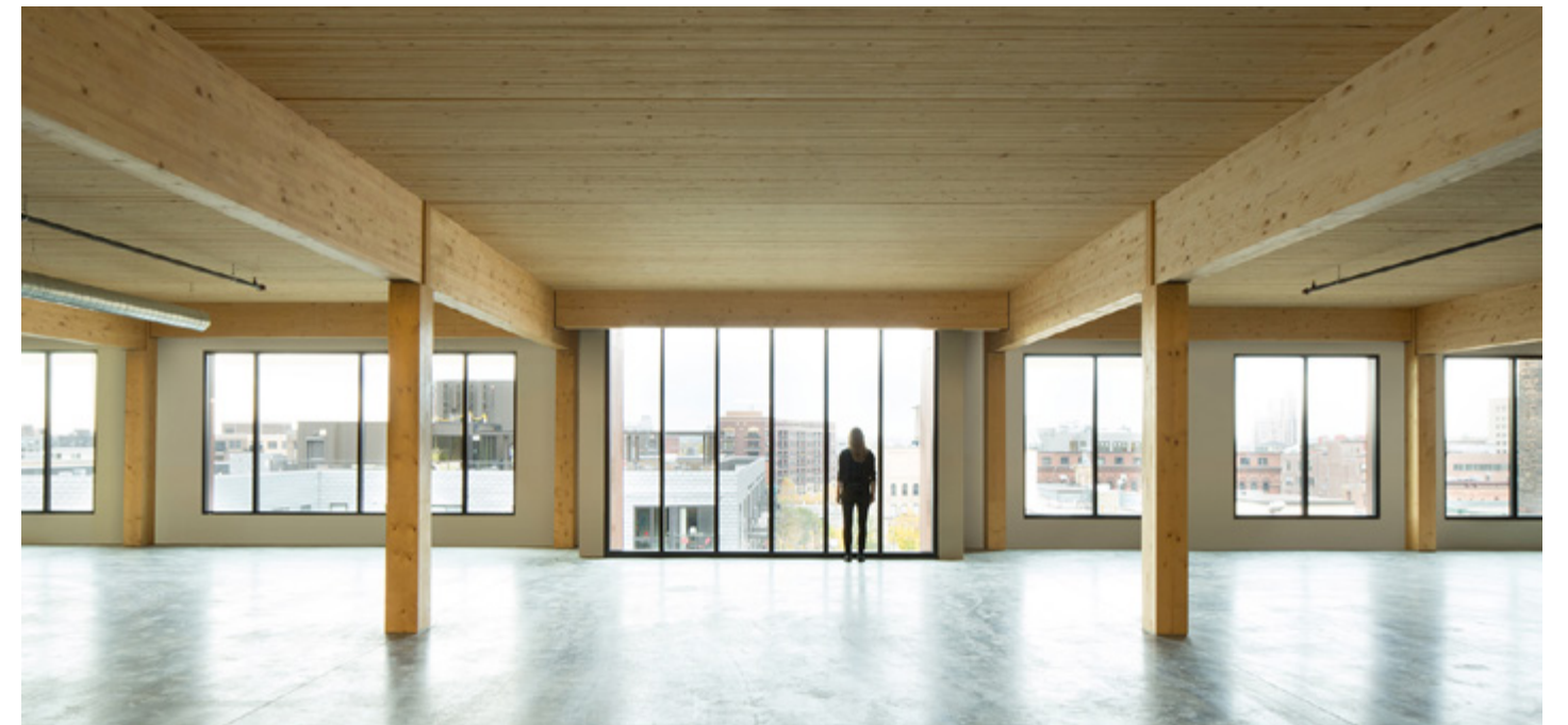
The T3 project in Minneapolis, Minnesota is a seven-storey, commercial building. Post and beam glulam frame with nail laminated timber (NLT) panels recreate the ambience of 19 th century brick and beam buildings. (Michael Green Architecture)
