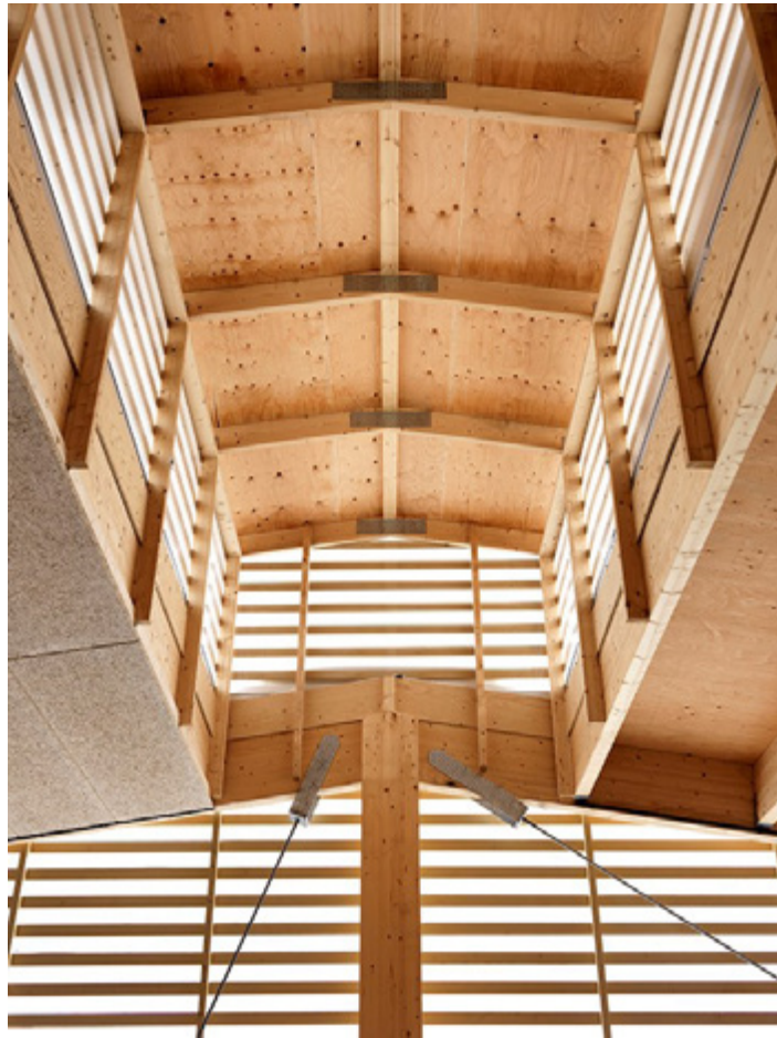
Four storey mass timber post and beam mixed use building. Located in Skellefteå, Sweden, this building features three storeys of parking on top of the ground level stores. The parking deck floors are covered with polyurethane to protect the cross-laminated timber decking from absorbing water. Generous overhangs and an open screen façade for ventilation ensure the drying potential exceeds the wetting potential on an annual basis to maintain a safe moisture balance. (Setra Group)
