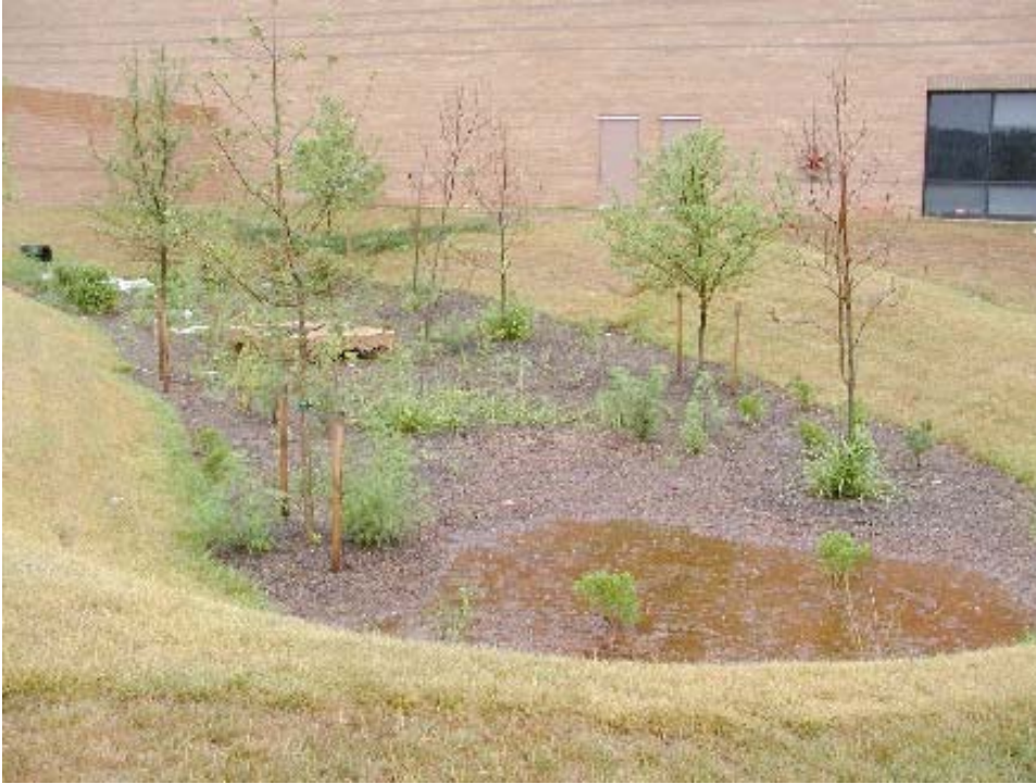
Figure 29. Water accumulations normally subside within hours of a storm's passage, and in rare instances may have a duration of one or several days.
