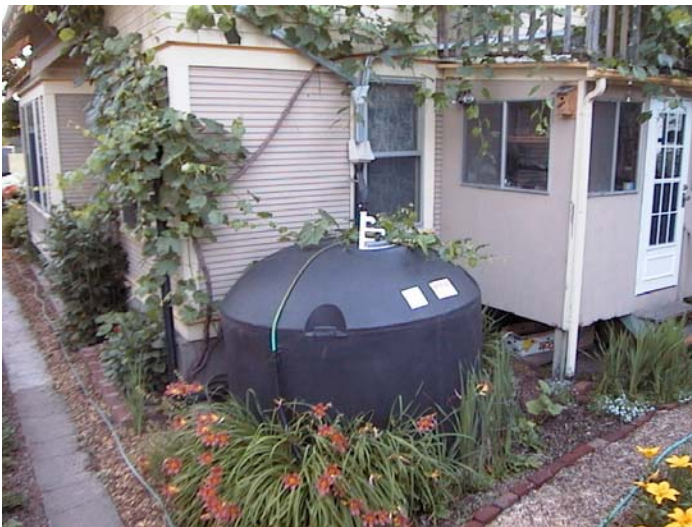
Figure 10. Cistern (1,500 gallon capacity) installed in Portland, Oregon and approved in 1998 for potable water use after treatment indicates the future of downspout disconnection.
