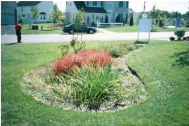
Figure 35. Bioretention cell accepts runoff from roadway for temporary storage and filtration during storm events.
