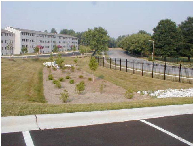
Figure 26. A newly constructed detention basin that will eventually mature into a tree filled meadow.
