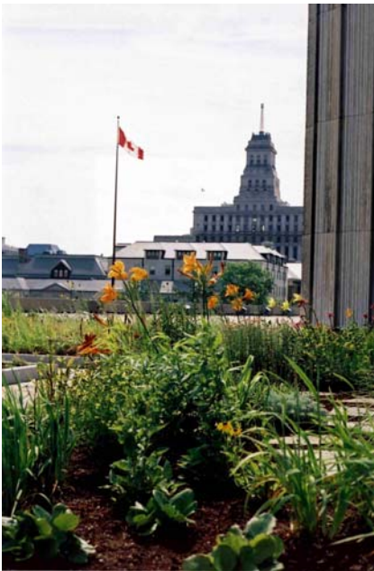
Figure 22. Green roof demonstration project at Toronto City Hall transforms dull concrete into a verdant landscape while reducing cooling loads and stormwater runoff.
