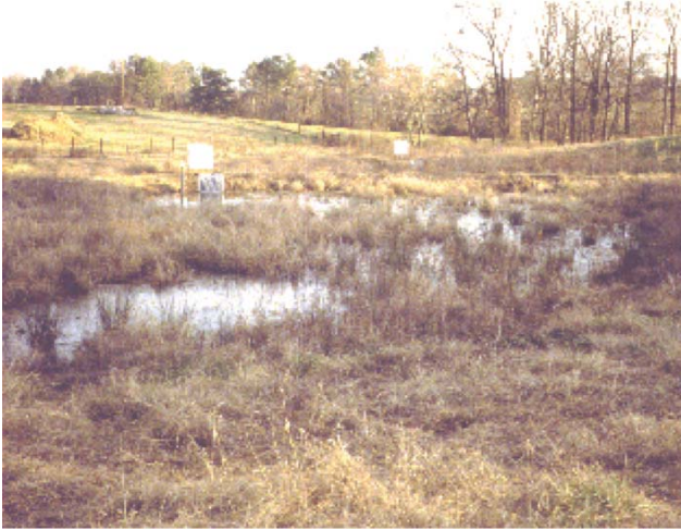
Figure 20. Retention basins of the kind shown in this figure are becoming less popular due to concerns for mosquito breeding grounds that may spread the West Nile virus.
