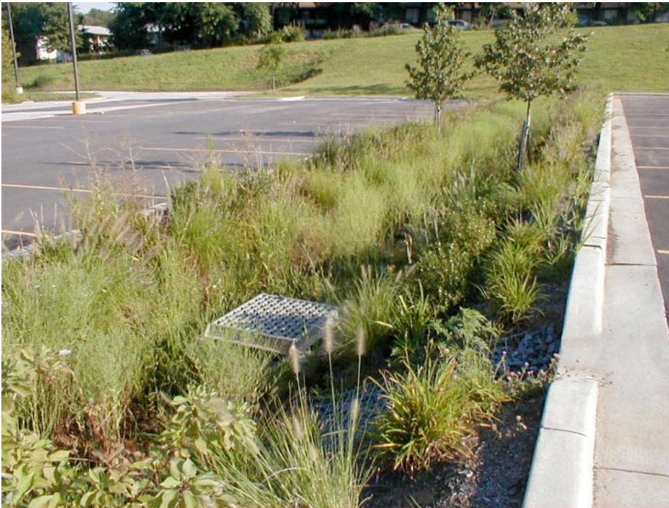
Figure 36. Bioretention strips may be integrated within parking lots to reduce runoff and effectively filter road de-icing salts. Note the incorporation of a catchbasin to capture extreme weather flows and avoid local water accumulations.
