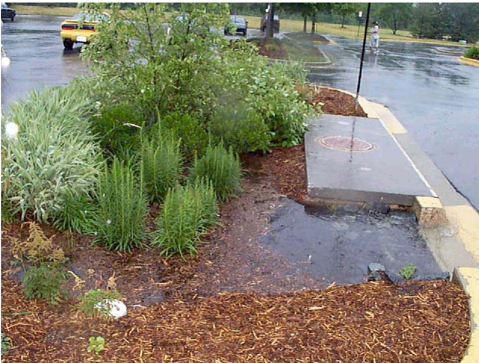
Figure 37. An example of a bioretention cell integrated within an existing parking lot.
