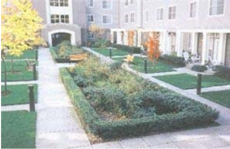
Figure 34. Courtyards and perimeter yards may be used to advantage, directing runoff from roofs and paved surfaces to bioretention cells that incorporate plantings.
