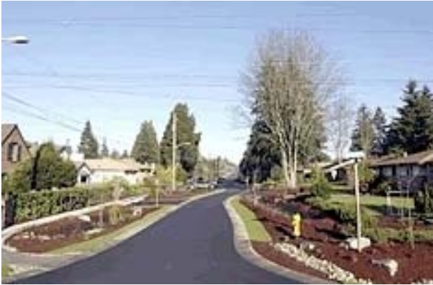
Figure 33. Bioretention cells may be cost effectively incorporated into existing developments when these are being re-paved or improved.
