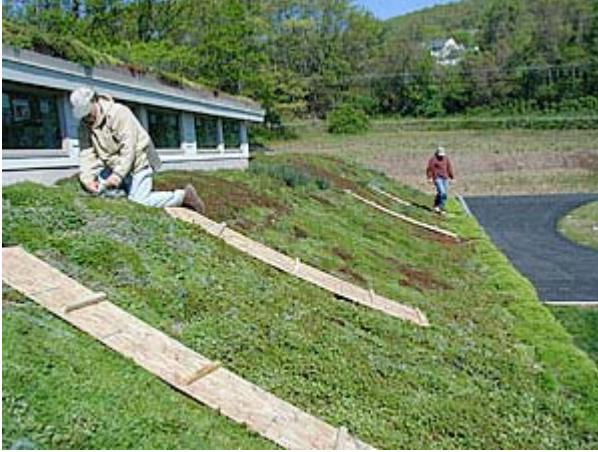
Figure 23. Green roofing technology improves energy efficiency and extends the life roofing membranes by protecting them from exposure to sunlight and temperature extremes. These benefits more than offset the initial cost premium associated with green roofs.
