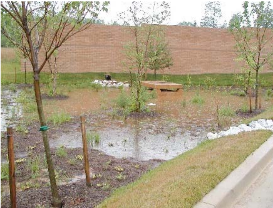
Figure 28. Flood tolerant tree species must be selected for use in detention basins. Local varieties that thrive along lake shores and stream beds are reliable choices.
