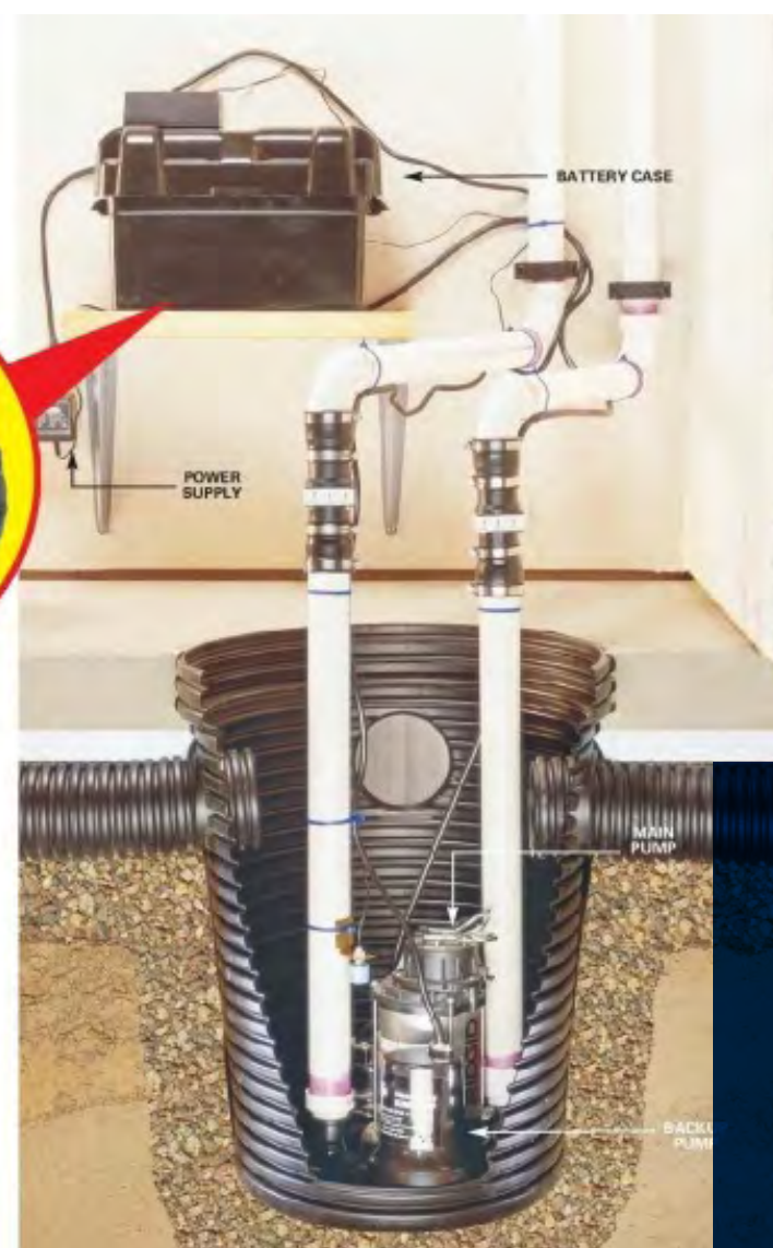
Providing a second battery powered sump pump is now widely recognized as a prudent redundancy measure to prevent basement flooding when power outages and extreme rainstorms coincide, or when the main sump pump fails.
