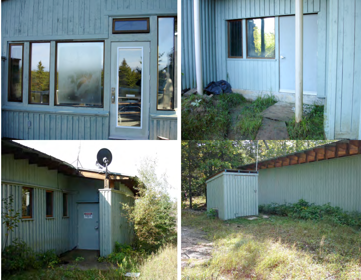
Figure 7. Some of the glazing unit seals have failed indicating interstitial condensation and the need for replacement (top left). The wood siding is beginning to indicate signs of weathering and should be refinished within the next few years to avoid deterioration of the wood. Permanent ramps and/or paving needed at lower level door (top right) and battery/mechanical room (bottom left). Generator shed (bottom right) is in good condition and a photovoltaic panel has been mounted on a pole to maintain charge of the generator's starter battery. 2010.
