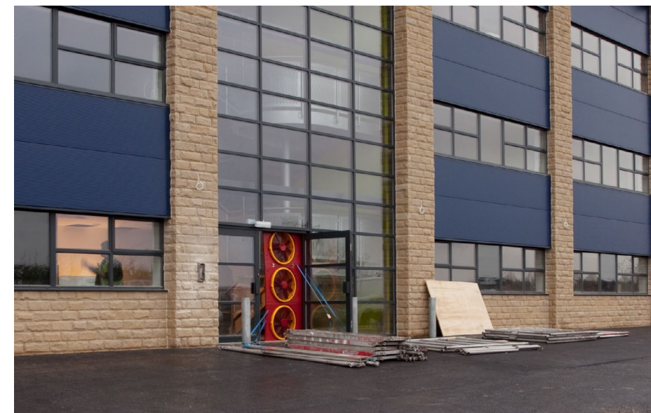
Fan depressurization testing of a commercial building air barrier system is an essential part of building envelope commissioning. By observing best practices for building envelope commissioning, it is possible to avoid discovering unsatisfactory performance after it cannot be easily remediated.
