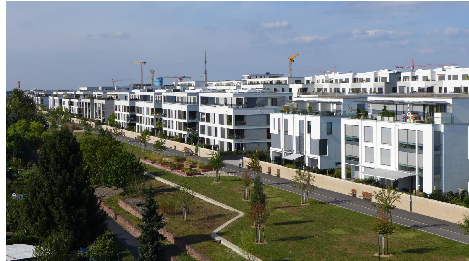
Passive measures help address sustainable development and climate change mitigation imperatives. In a new city district of 116 hectares, the Bahnstadt Project in Heidelberg, Germany is being constructed to the Passive House Standard and is serviced by a renewable district energy system for satisfying thermal and electrical loads. [Photo: C40.org]
