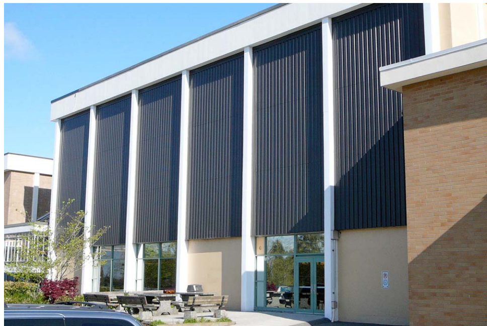
Figure 34. Example of solar air heating panels attached to south facing wall of a high school. [Photo courtesy Conservall Engineering]
