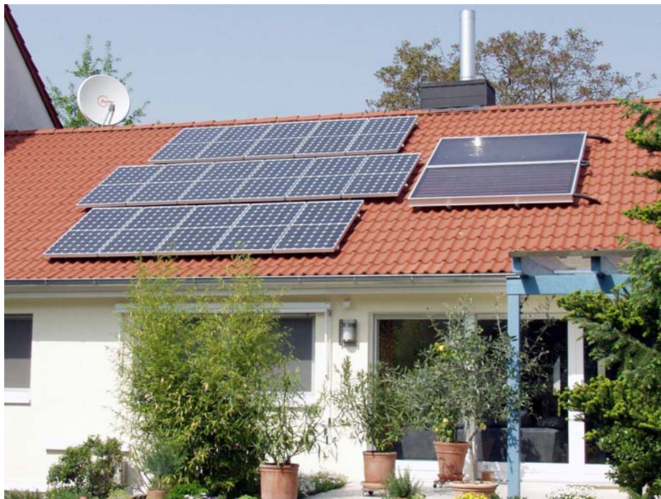
Figure 32. PV technology and solar water heaters are common in European housing where large subsidies have been made available to homeowners for their installation. Note the inclusion of biomass space heating. [Photo courtesy International Energy Agency]
