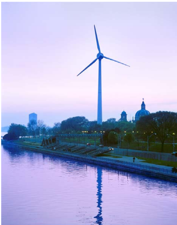
Figure 41. 750 kW wind turbine at Canadian National Exhibition site in Toronto.
