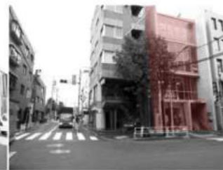
Redevelopment as commercial usage area in case of site subdivision without changes of usage of building.
