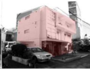
Redevelopment as commercial usage in case of integration of sites from residential use.
