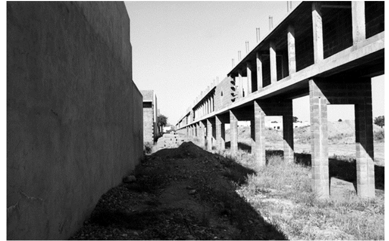
The new aqueduct under construction in 1980s (Source: The Architectural Review)
