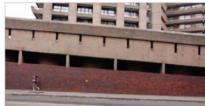
Blank frontage on Aldersgate Street
