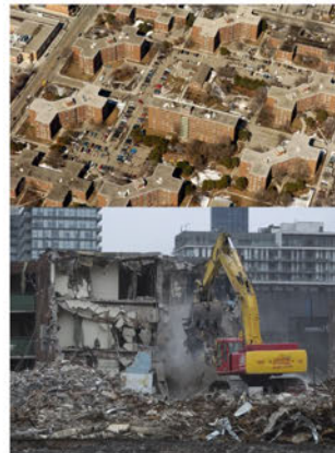
Regent Park social housing demolition for "revitalization" and new development
