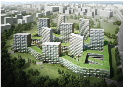
NINE DRAGON HOUSING COMPLEX (2011)
